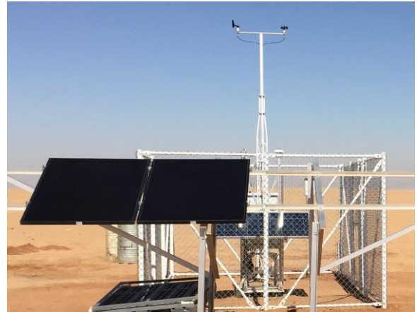
Fig. 5. Test modules and Station Enclosure High data acquisition sampling rates (10 secs) were applied to deliver 10 minutes averages for all relevant climatological and performance variables. The measurement campaign has started in January-2016 and will extend until June-2016.
