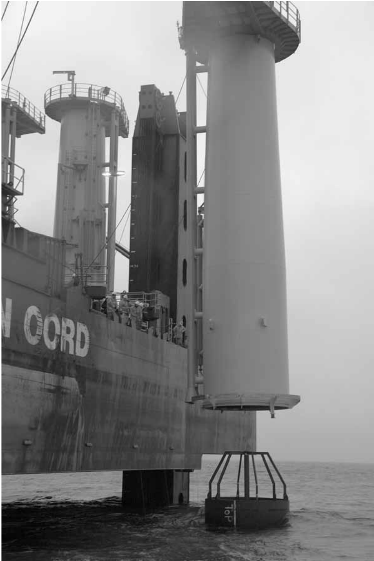
16.24 Transition piece installed by Van Oord at Q7, Prinses Amalia WP (© Van Oord Dredging & Marine Contractors).
