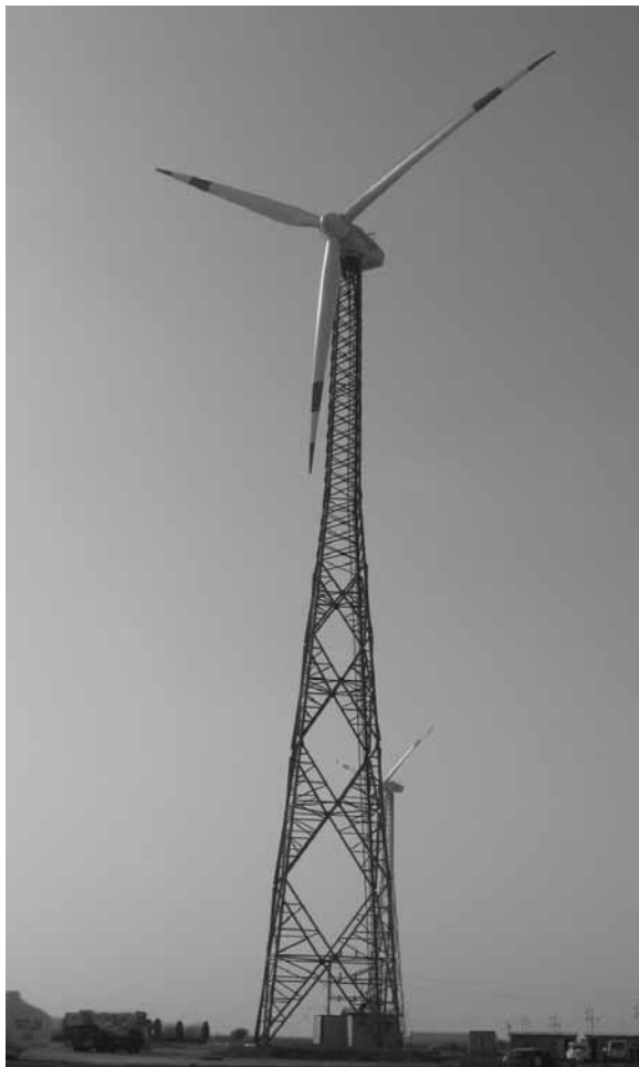
9.1 Lattice tower. Photo by Marcus Klose, Germanischer Lloyd.
