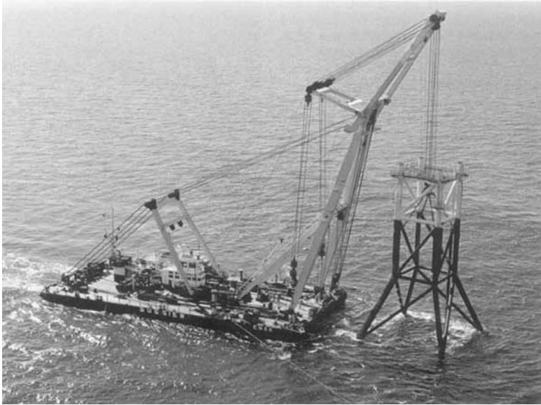
16.25 Positioning and sinking of a jacket using a floating crane (© F + Z Baugesellschaft mbH, Hamburg).
