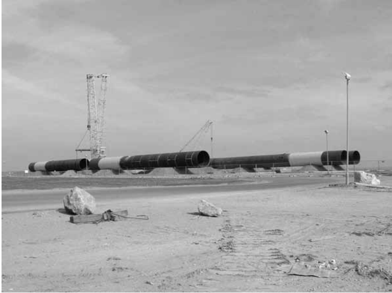
16.2 Monopiles for the North Hoyle wind farm (© RWE Innogy GmbH).
