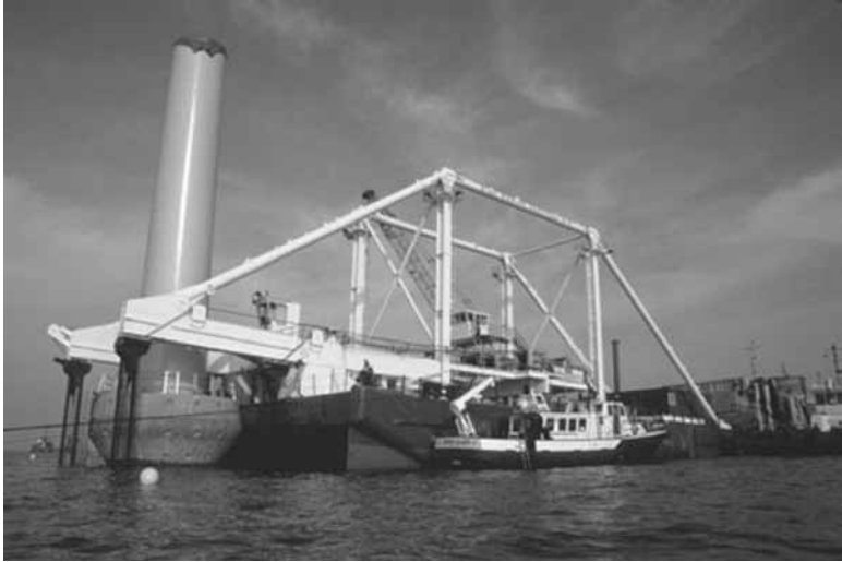
16.27 Transport of a gravity based foundation to the location of the offshore wind farm Middelgrunden (© Middelgrunden Wind Turbine Cooperative).
