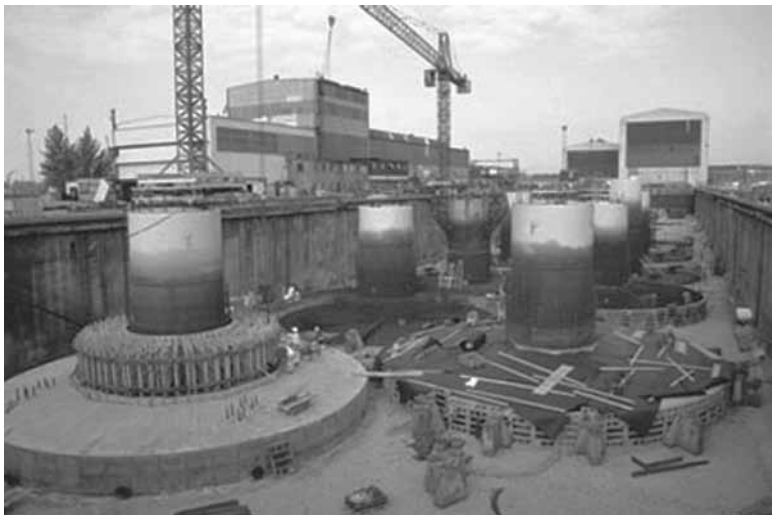
16.26 Construction of gravity based foundations for the offshore wind farm Middelgrunden in a dry dock (© Middelgrunden Wind Turbine Cooperative).
