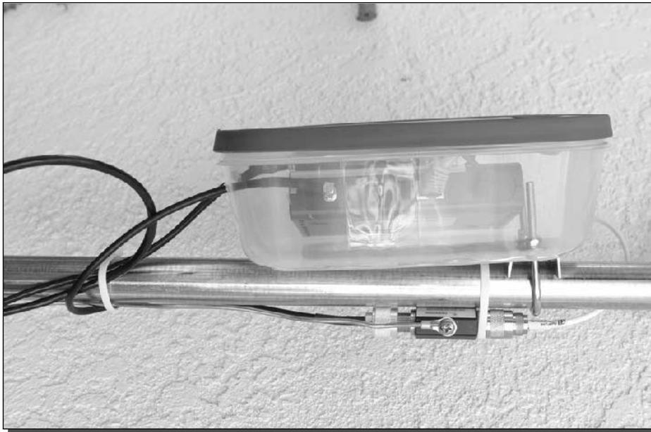
FIGURE 8-19: Placement of the lightning protector on the pole.
