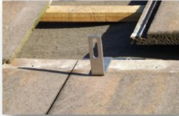
To install solar panels onto an existing tiled roof, individual tiles are slid out and a roof hook is fitted beneath the tile, mounting directly onto the underlying roof truss. Once mounted, the original tile can be slid back into position. Depending on the type of tile and the roof hook design, it may be necessary to chisel out part of the underside of the tile in order to achieve a good fit.
