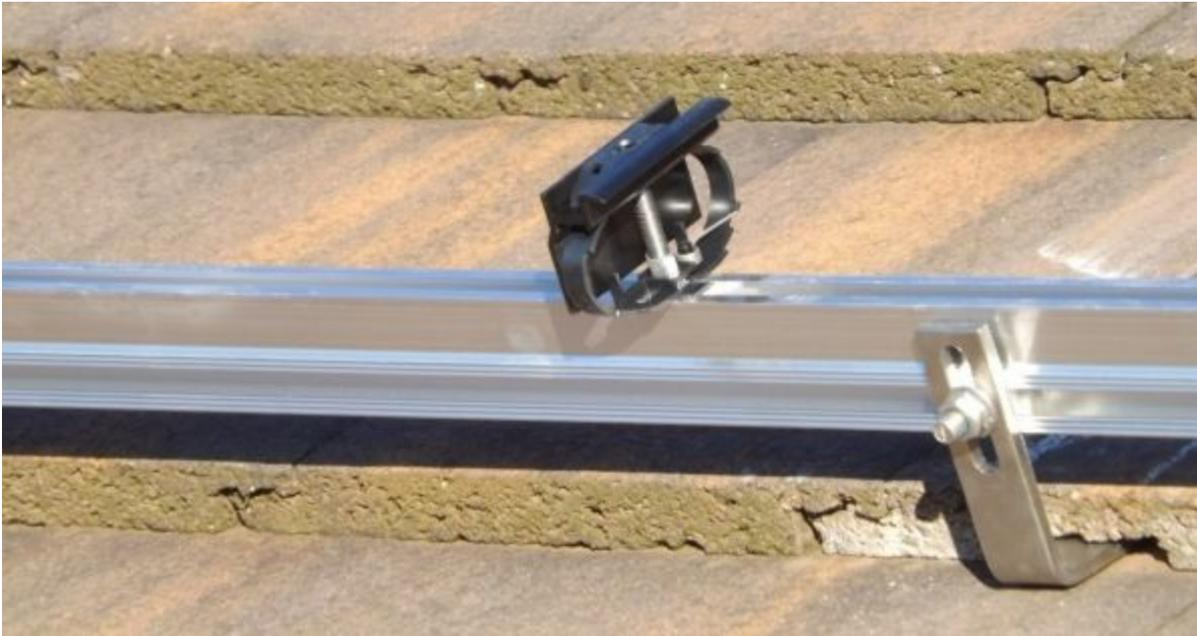
Finally, the first solar panel can be fitted into position. Four clamps are used to hold a solar panel into position. However, each clamp can hold two solar panels down when the panels are next to each other.
